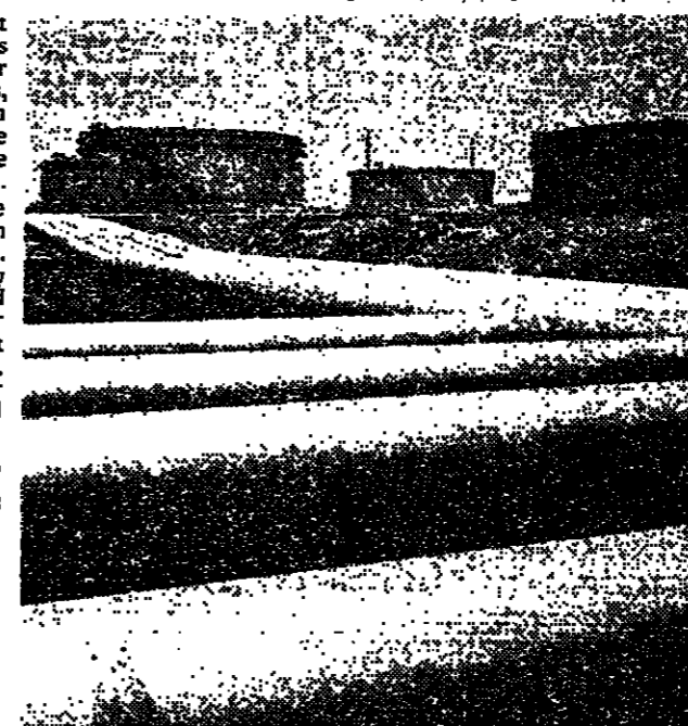
Pipes and storage tanks near a petrochemical plant on Kharg island.
